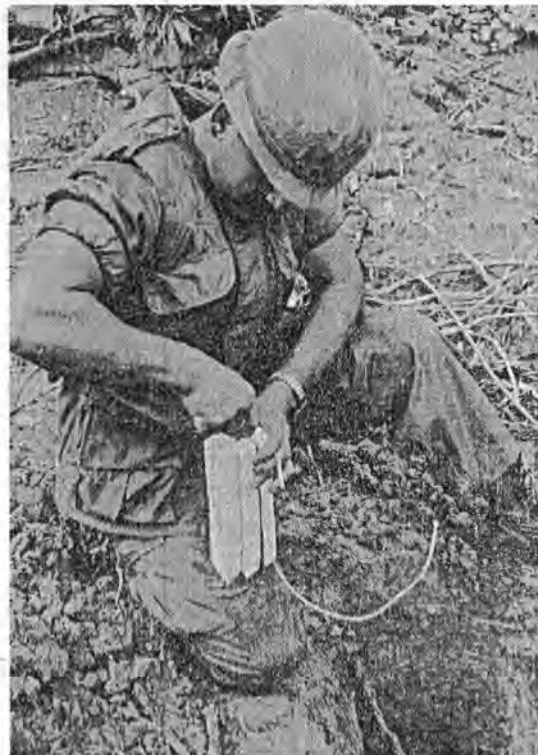
DESTROYING TROUBLE—Staff Sergeant Obel D. Nazario-Almodovar of Company C, 4th Combat Engineers prepares a charge to destroy a Viet Cong mine.
